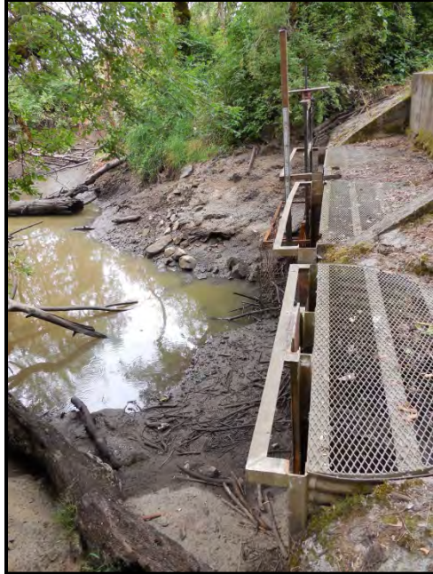
Photo C-3 Upstream end of one of the hydraulic control structures at Multnomah Marsh.
