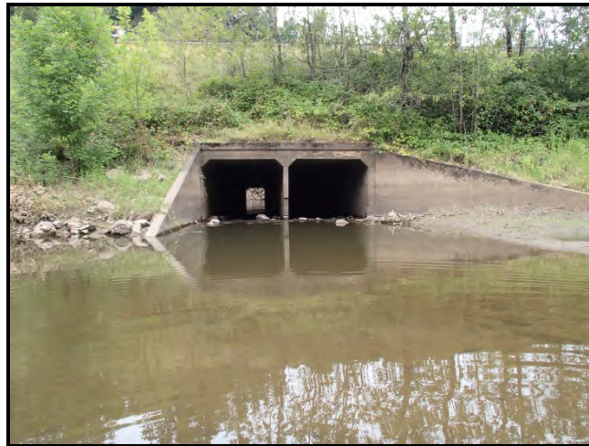
Photo C-4 View of twin box culverts at downstream end of Mirror Lake.
