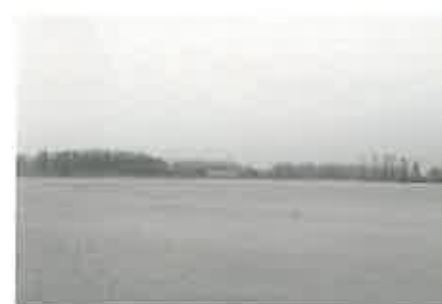
(E) Holding Pond & Facilities
